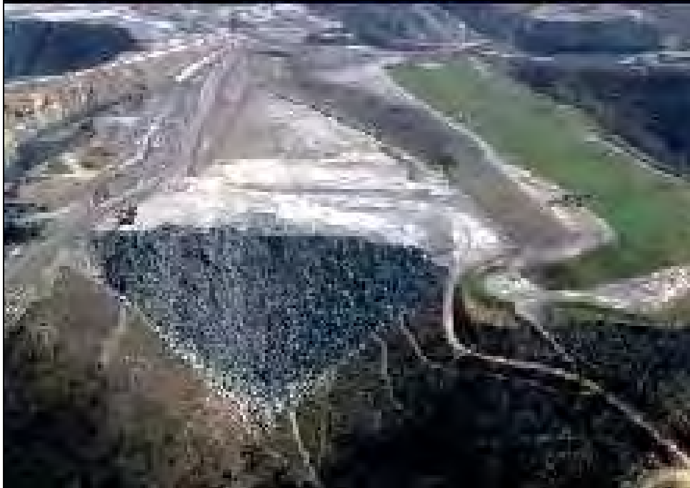
Figure 1-2. A VF in operation. The excess materials from a MTM operation are being placed in this adjacent valley.
